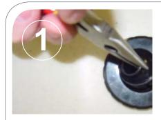
Remove the jet eyeball using the needle nose pliers.
